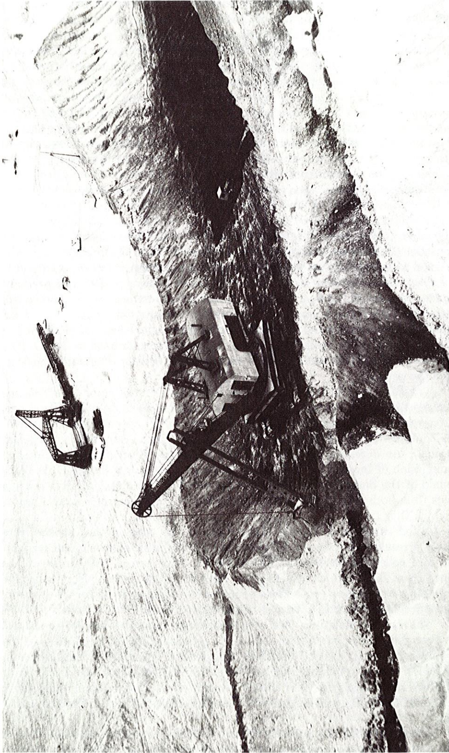
Strip mining with electric shovel, Western Dominion Coal Mines, Taylorton.
